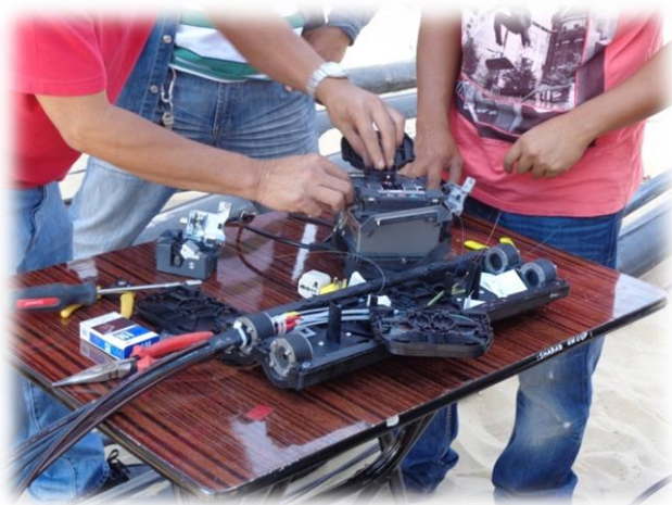
FOC Cable Splicing / Jointing Multimode Cables / Sensing Cables of 380kV
