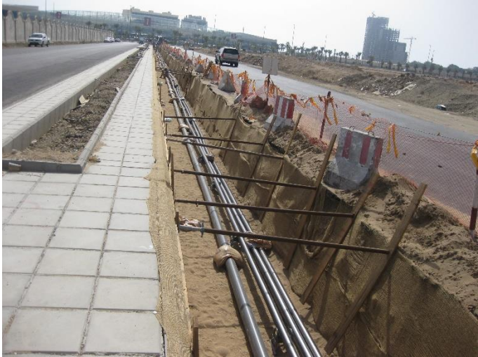
High Voltage Cable Pulling
