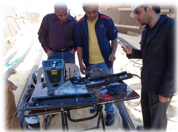
FOC Cable Splicing / Jointing Multimode Cables / Sensing Cables of 380kV
