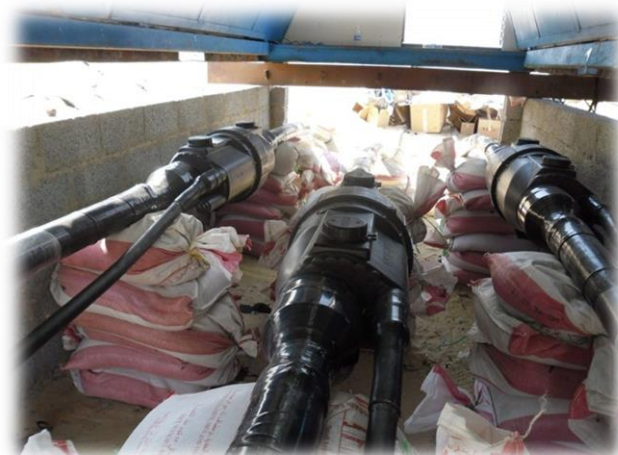
115kV EHV Cable Jointing Pfisterer Joints MSA145
