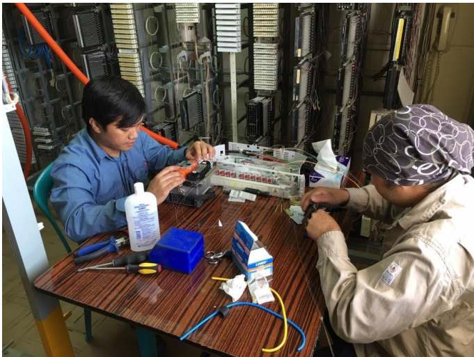
Fiber Optic Cable Splicing Testing & Commissioning
