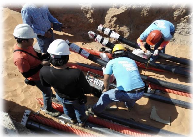
10kV DC Sheath Testing on Outer Sheath Applied After Cable Laying
