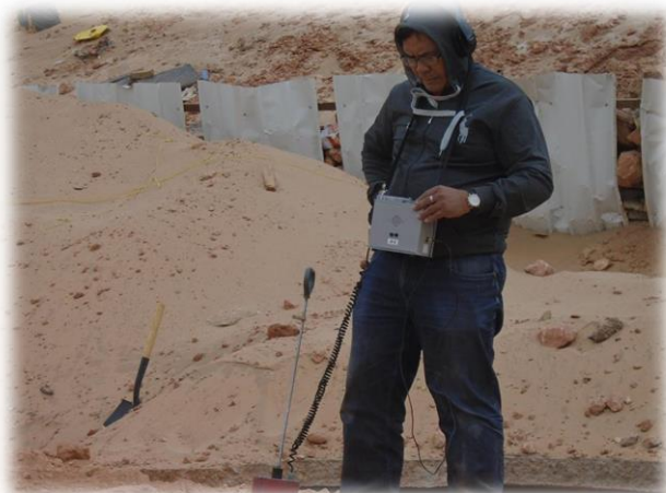
Cable Fault Location Contractor: Hadi Haider Contracting
