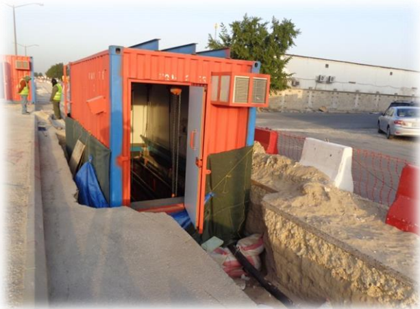
115kV EHV Cable Jointing
