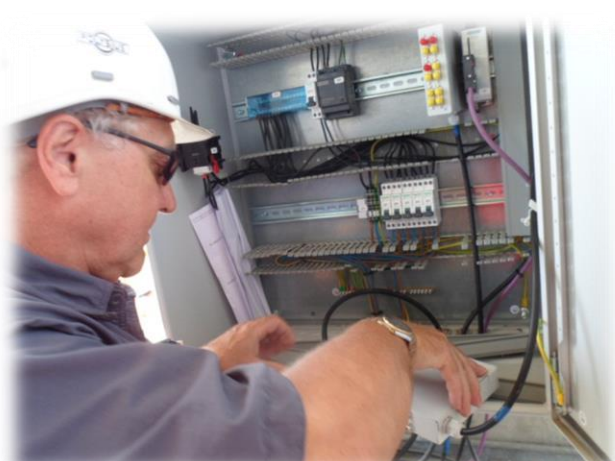
FOC Testing Tabuk Cement Contractor: Thyssen Krupp / Uhde Arabia
