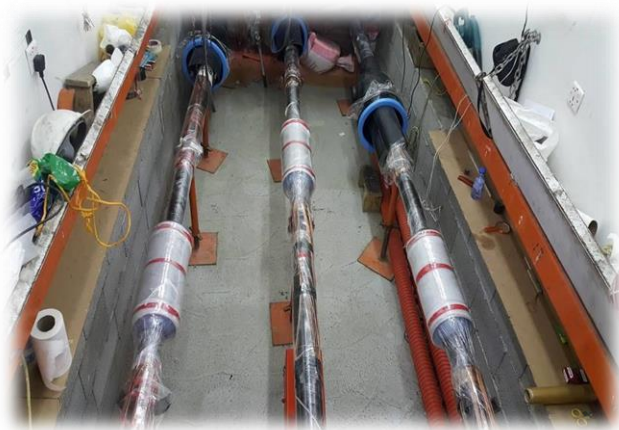
132kV EHV Cable Jointing MSA 145 PFISTER Made
