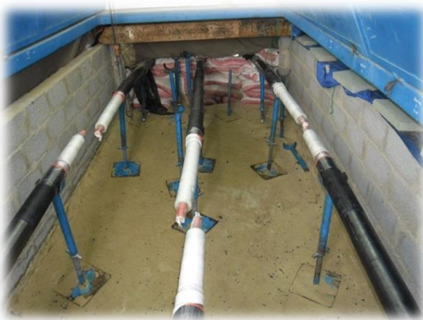
115kV EHV Cable Jointing
