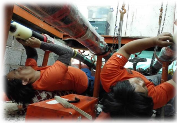
115kV EHV Cable Jointing MSA 145 PFISTER Made
