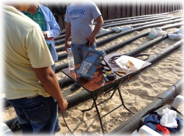
FOC Termination Post Installation Testing Multimode Cables / Sensing Cables of 380kV
