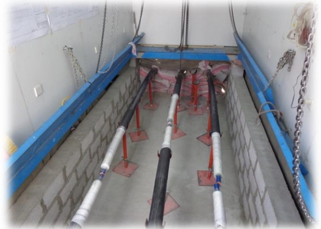
115kV EHV Cable Jointing
